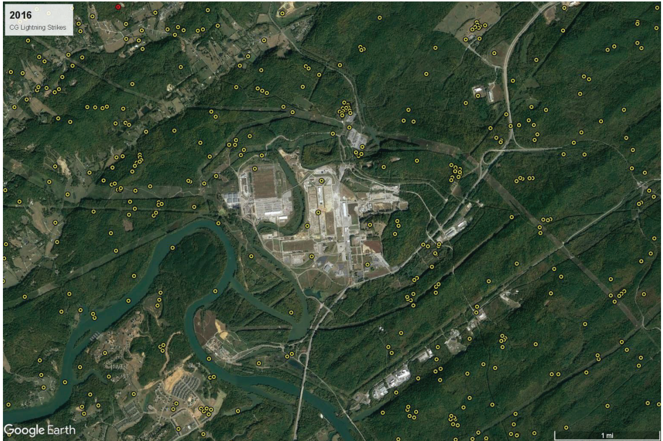
Figure 3-9: Lightning strikes recorded at or near ETPP during 2016
